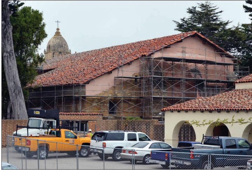
Contractors erected scaffolding this week in preparation for removing roof tiles and drilling into the walls of the Carmel Mission Basilica to strengthen them in a \$5 million seismic upgrade project. The work is being funded by the Carmel Mission Foundation, which is still seeking donations for other improvements at the historic Mission that was completed in 1793.
